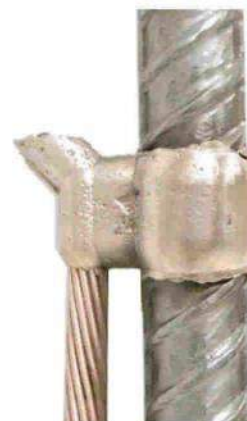
• 95 mm² Copper Cable to 40 mm Rebar
